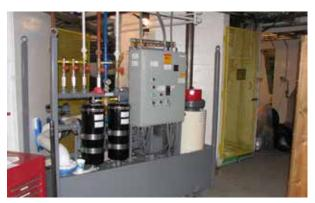
New LE-designed lube system installed and running.
