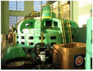
275-gallon tote and filter cart that was used to transfer the turbine oil into the turbine.
